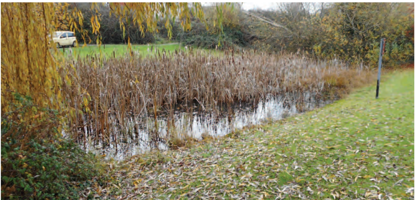
Figure 6: SUDS schemes are now common in best-practice housing development.
