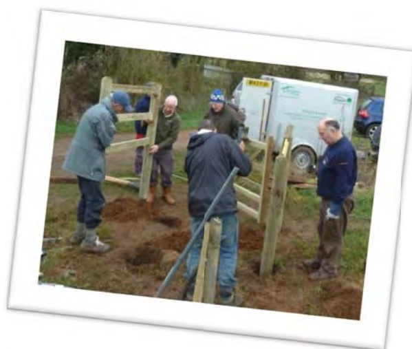
Volunteers installing gate ( Howard Dell)
