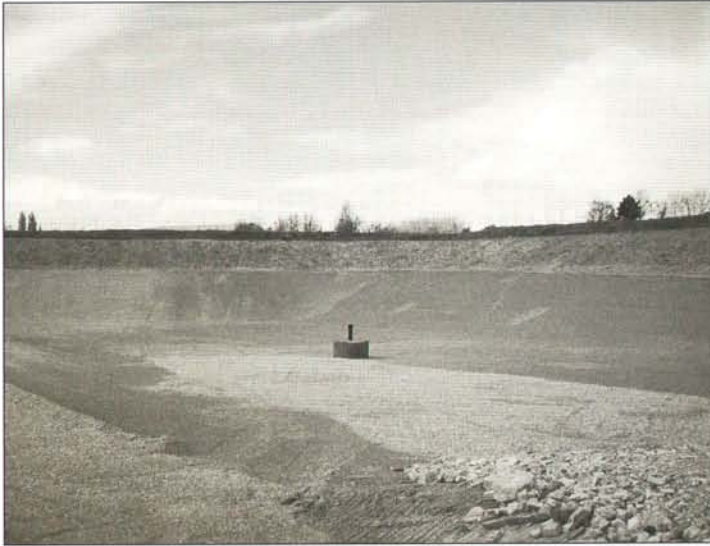
Clay cell in preparation for waste disposal at Dix Pit
