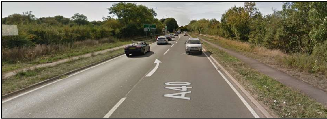
Figure 3-6 A40 Footway/Cycleway between Eynsham and Cassington
