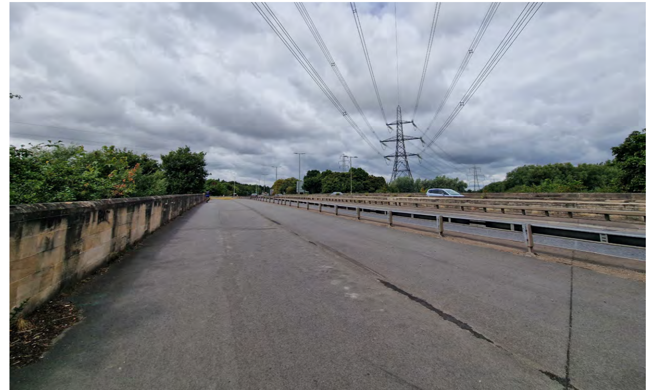
Existing Kennington rail bridge (photo taken Summer 2021)
