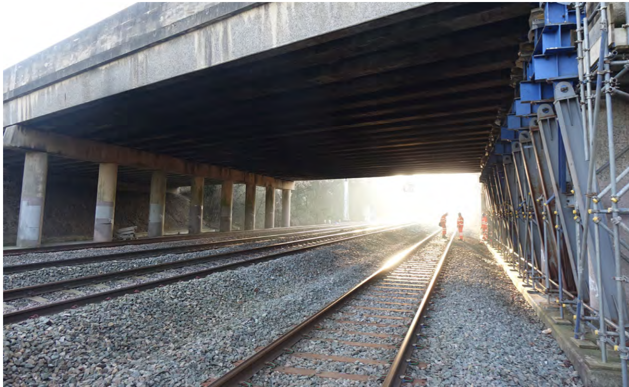
Existing Kennington rail bridge (photo taken Summer 2021)
