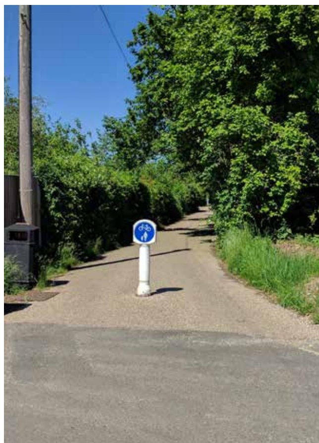
Placement of a single bollard to prevent vehicles from entering the cycle path
